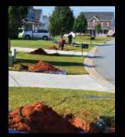
Cable/Telecom — Stitch boring with the Hole Hammer is a costeffective method to install highproduction cable and telecom projects in finished landscapes.
