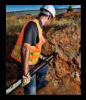
Electric — Hole Hammer has the punch you need to power through difficult ground conditions when installing electric upgrades and drops.
